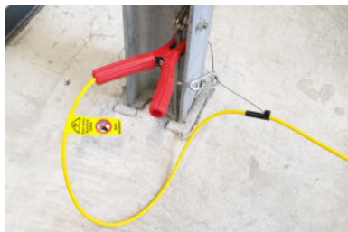
Earthing at the foundation earth
