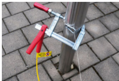
Earthing on a mast with the help of a screw clamp
